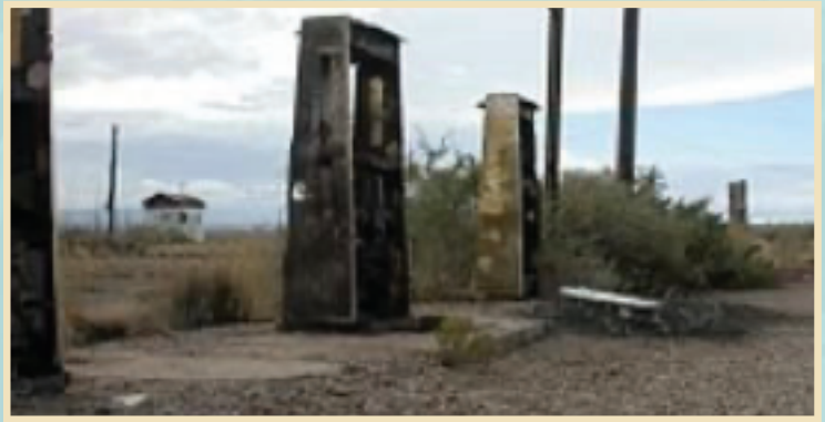
Abandoned Gas Pump Island, photo: Wikipedia.org
